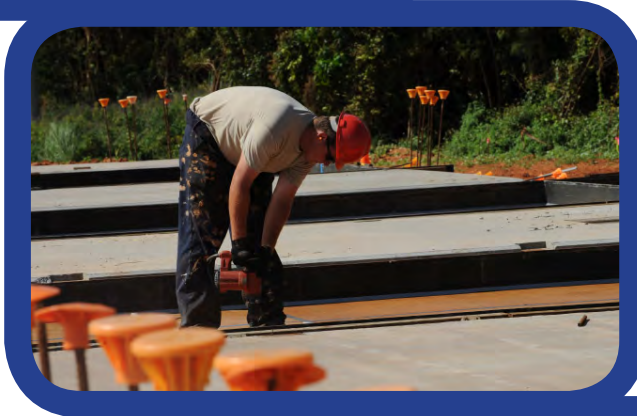
U.S. Air Force personnel perform construction at the Northwest Field site on Andersen Air Force Base, Guam, January 2009
